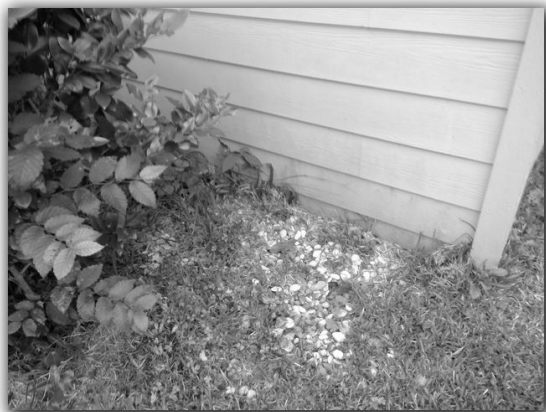
front right side and west wall in front Inadequate grading clearance to exterior wall surface
