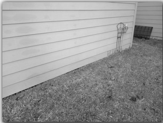
front right side and west wall in front Inadequate grading clearance to exterior wall surface
